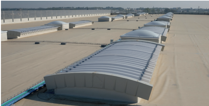
Tetto piano con supporto in PVC. Deck roof made with PVC film.
